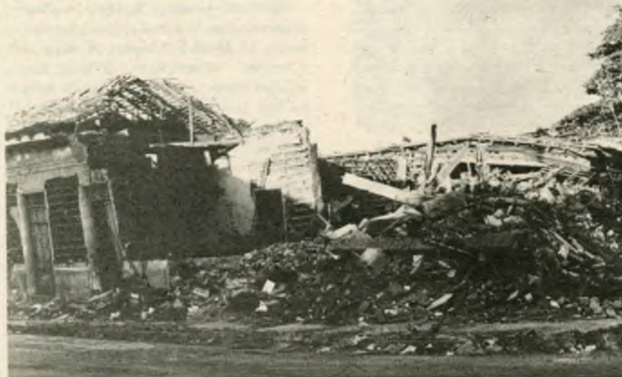
Destroyed buildings like this line every block.
